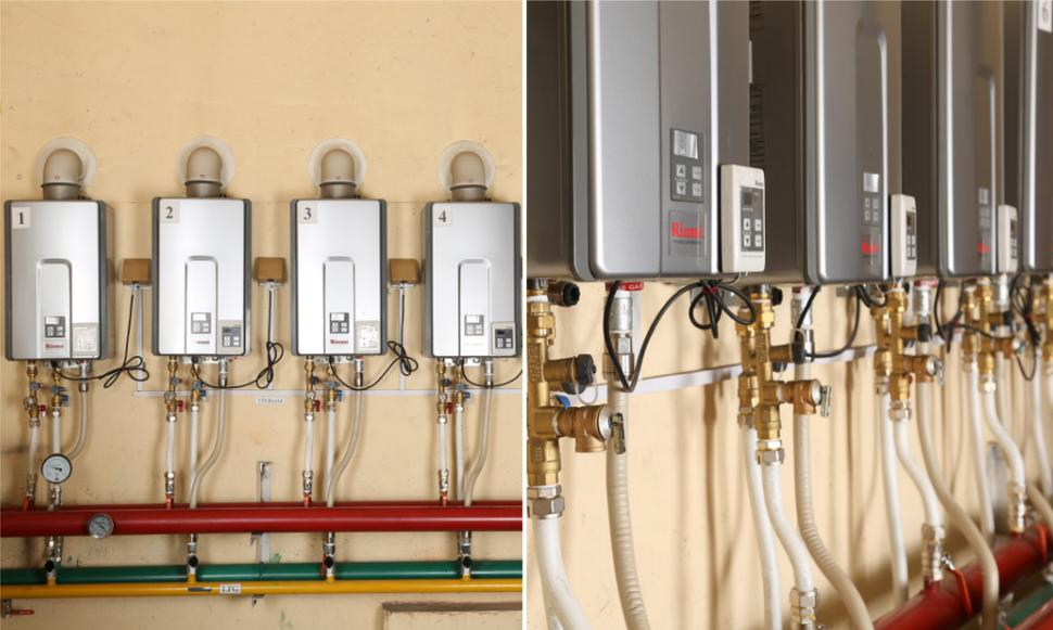
**“ As of November 2020, gas heating has been successfully installed in 11 state-owned schools, kindergartens, and offices located in the capital city. By converting these facilities to gas heating, we were able to eliminate 2,394 tons of raw coal used per year, 6,387 tons of CO2, and 511 tons of ash and dust. Now, 1,760 students and 437 employees have clean air to breathe, and can be educated and work in a healthy and comfortable environment.**
